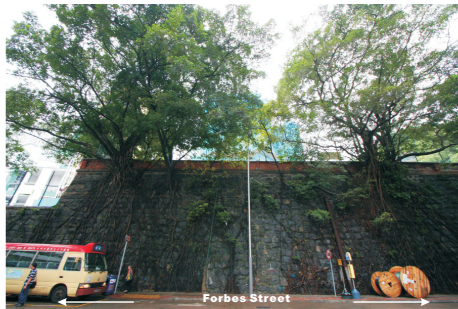
LR1.2 Wall Trees At Forbes Street Temporary Playground
