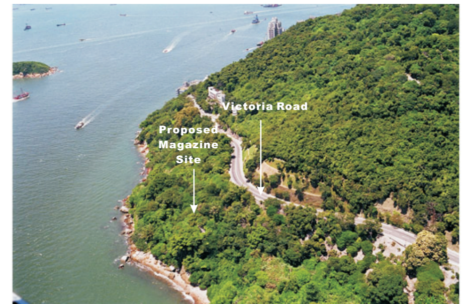
LR2.1 Roadside Planting along Victoria Road in Magazine Site
